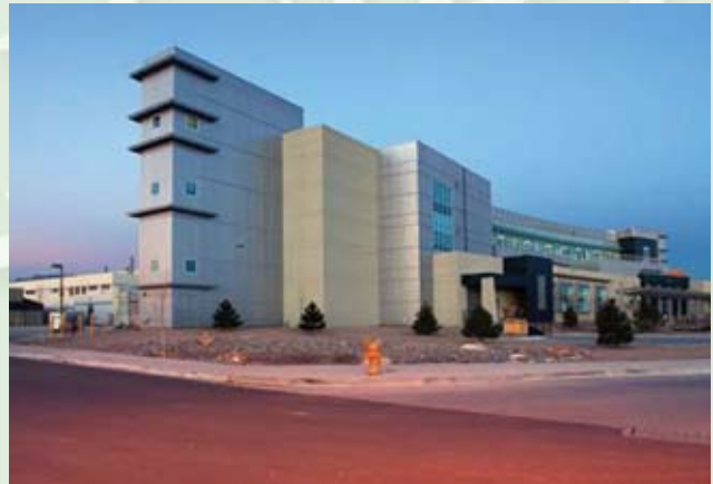
Southwest Elevation of JCEL
