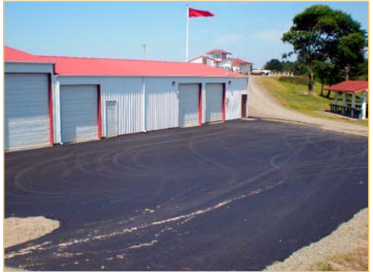
Completed engineered cap over former landfill at MARF Range Maintenance Building, Camp Rilea.
