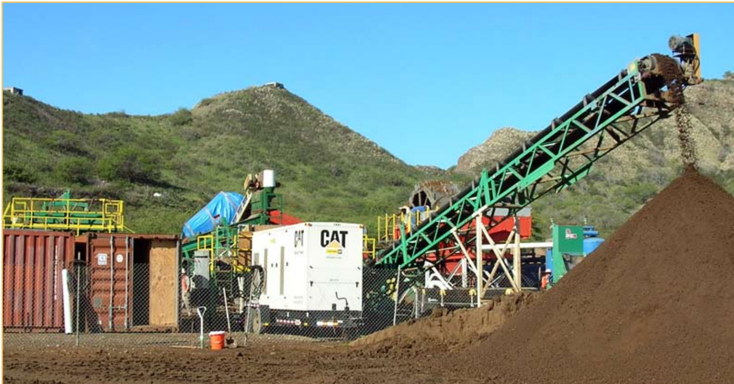
The contractors working on the processing equipment. Notice the cleaned and processed soil falling from the conveyor belt. Also notice the pillbox located on the rim of the crater.
