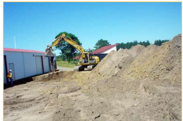
Landfill debris is removed from the Camp Rilea restoration site.
