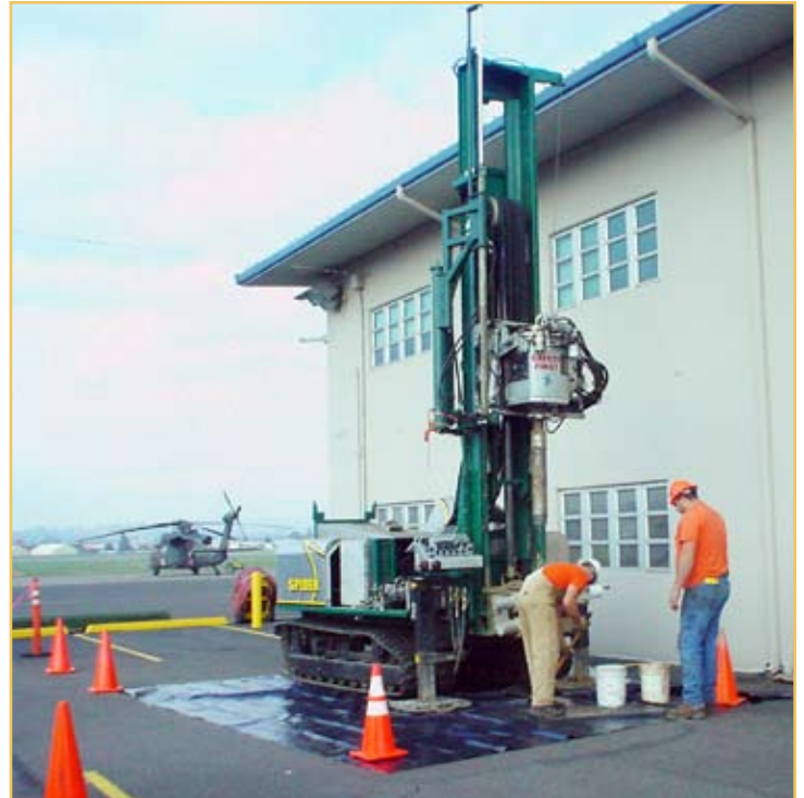
Drilling contractors installing groundwater monitoring well for vapor intrusion assessment use a limited access sonic drilling rig adjacent to active flight line at Army Aviation Support Facility #1.
