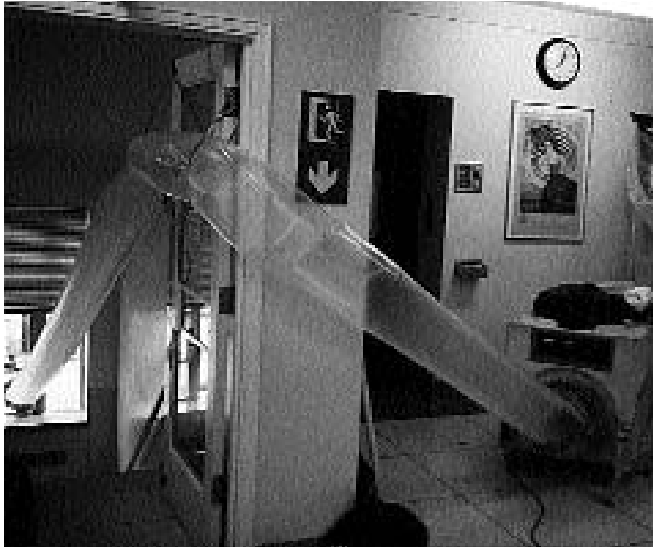
An air filtration device used to remove asbestos during an asbestos abatement project in Toronto
