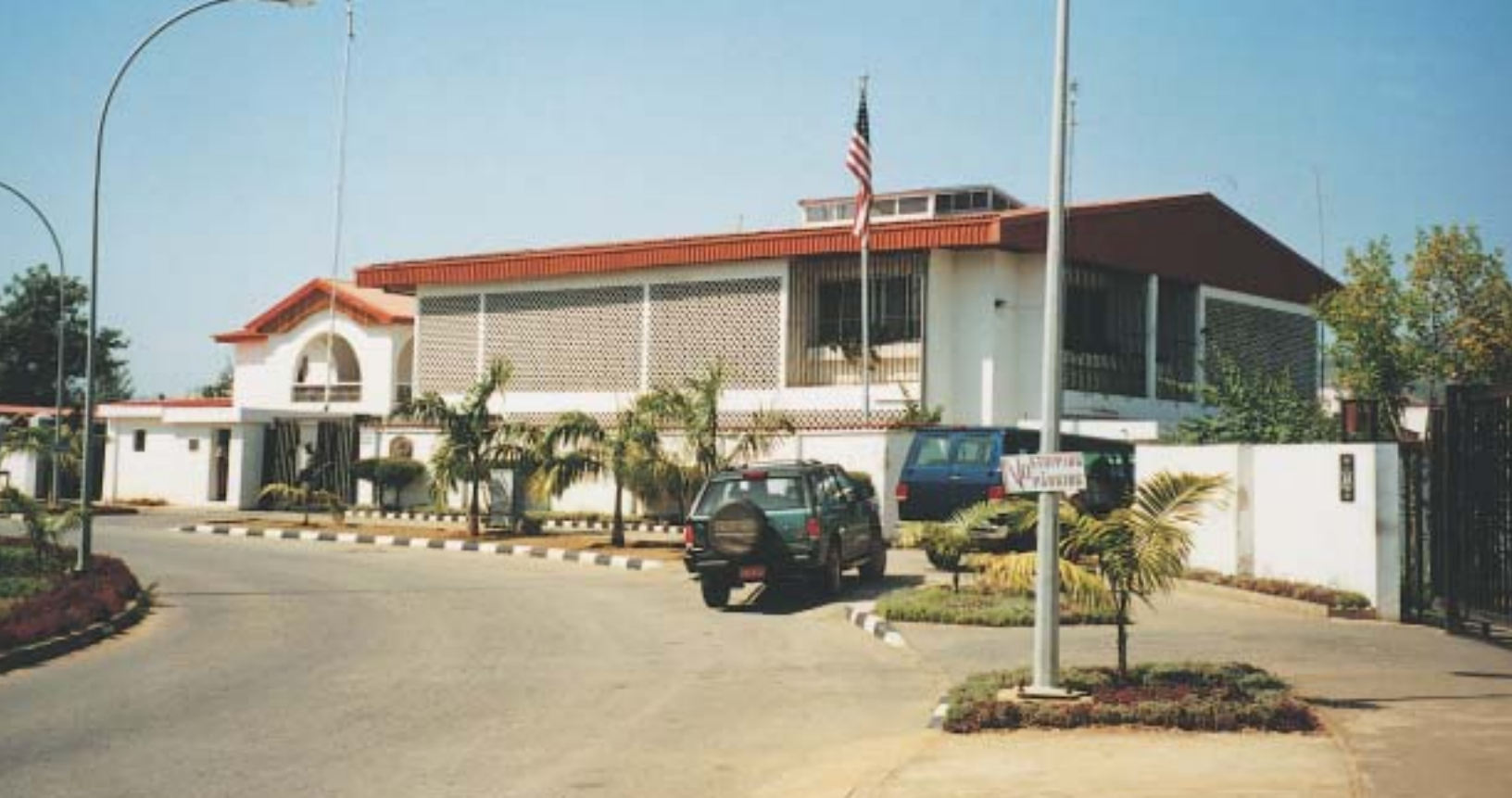
Above, the U.S. Embassy Office in Abuja. Below, a contractor, far left, briefs officers, from left, Alan Eyre, Richard Kaminski and John Bauman on the status of National Assembly construction.
