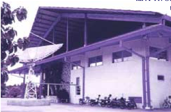
BBG transmitting station in Bangkok, Thailand.
