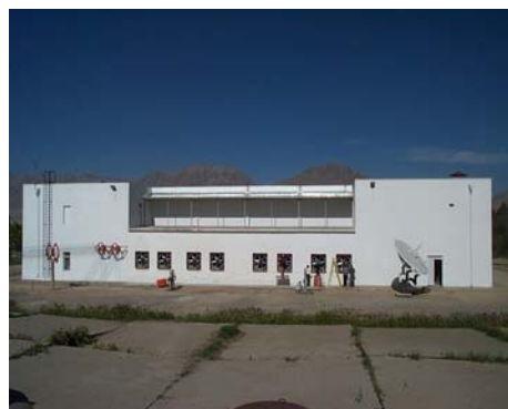
Figure 3 : Transmitting station after repairs by BBG
