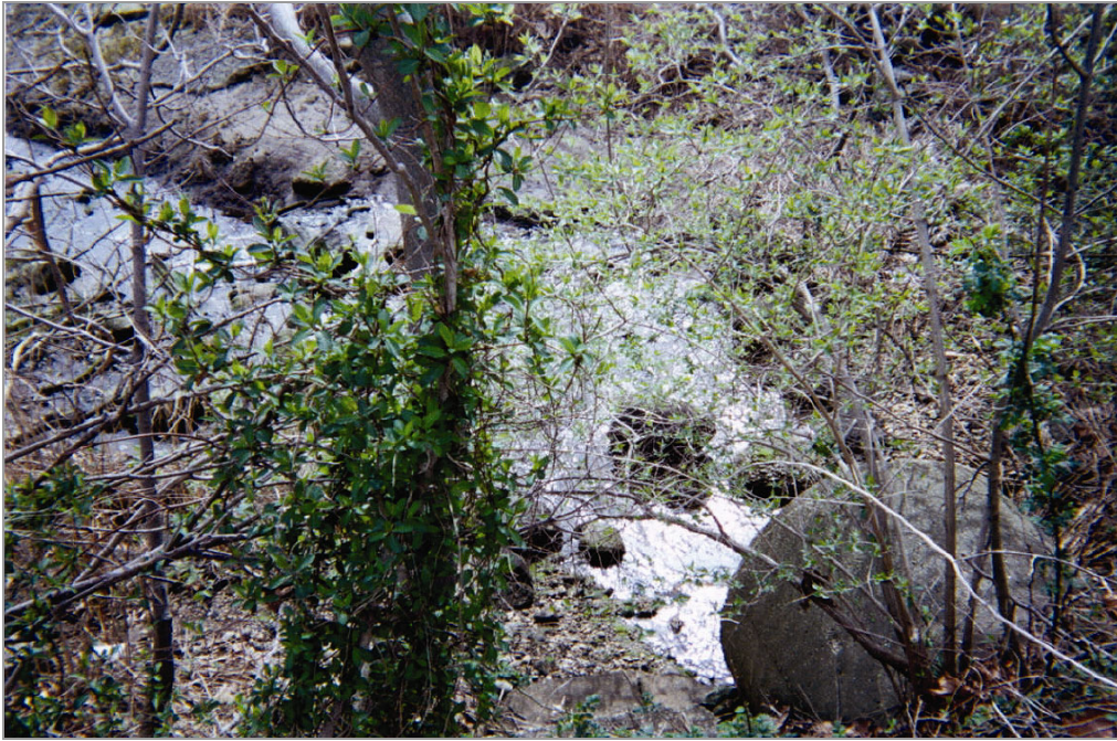
Photograph 15: The 24' stormwater outfall that discharges into the Bar Beach Lagoon that runs under Shore Road and the trail way discharges into the lagoon once it enters the lagoon. This photograph was taken at low tide in the lagoon and on a clear non-rainy day, thus the outfall appears to have a continuous discharge. The discharge appears to have created the channels that meander throughout the tidal flats. The County, according to Denise Herrington of the town of North Hempstead, apparently owns the outfall.
