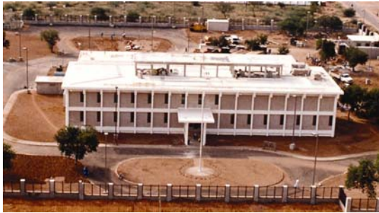
Exterior of Embassy Gaborone Chancery
