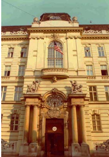
Exterior of Embassy Vienna
