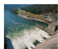
storms that generally carry the greatest flood risk. Drawing some water from the reservoirs allows more room to store rainfall and hold back floodwaters. This system prevents an annual average of \$224 million in flood damage and has saved an estimated \$5.7 billion since the dams were built.
