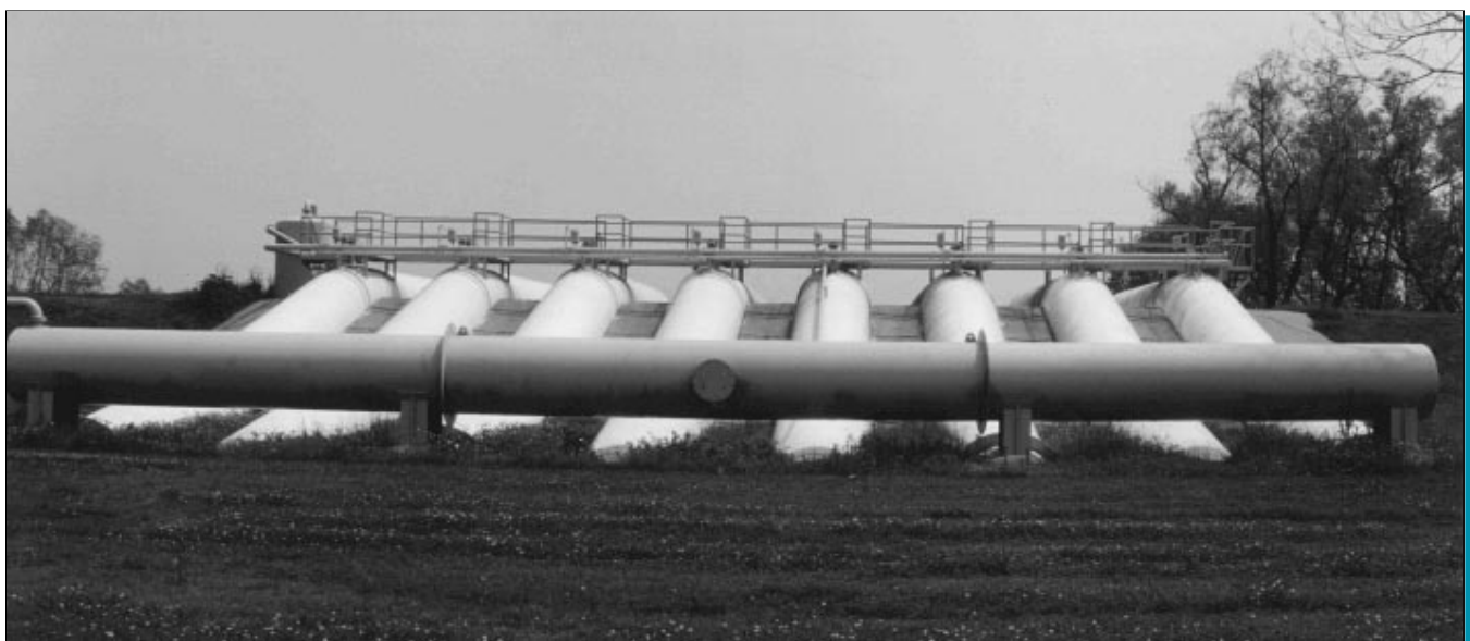
A view of the Naomi Siphon in Plaquemines Parish. Similar technology and structures will be used in the Myrtle Grove Siphon Project – one of two large-scale, freshwater diversion projects endorsed by the CWPPRA Task Force in February.
