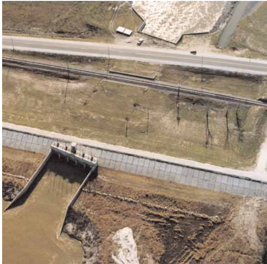
The rate of water flow through the Caernarvon structure can be adjusted to optimize benefits to the marshes.
