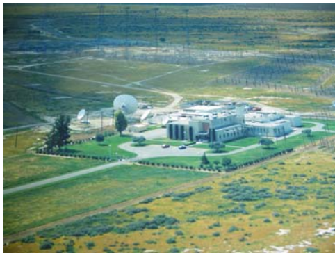
Aerial view of transmitting station
