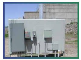
A NEWLY INSTALLED EQUIPMENT BOARD CONSOLIDATED JUNCTION BOXES, POWER PANELS, AND OTHER EQUIPMENT AT BROKEN BOW.
