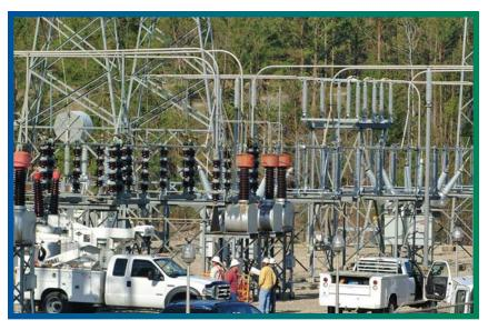
New renovations are distinguished in this photo by the color of insulator. The newer gray insulators on the right contrast with the brown insulators of the older equipment.
