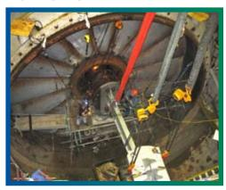
"The runner hub and shafts have been removed, and we're disassembling the wicket gate mechanism," says Beverly. "The next step is to remove the wicket gate ring, and then we'll proceed with painting and refurbishing the water passage."
