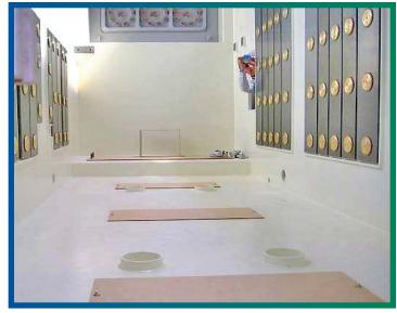
CARLOS VALENCIA EXAMINES THE INTERIOR OF ONE OF Norfork's new autotransformer tanks prior to the Installation of the windings.
