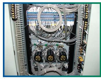
A NETWORK OF INTERIOR PANEL WIRING CONNECTS THE NEW PROTECTIVE RELAYS FOR CANNON'S UNIT # 2.
