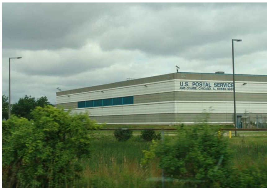
The Chicago AMC at Chicago’s O’Hare International Airport, June 5, 2007.
