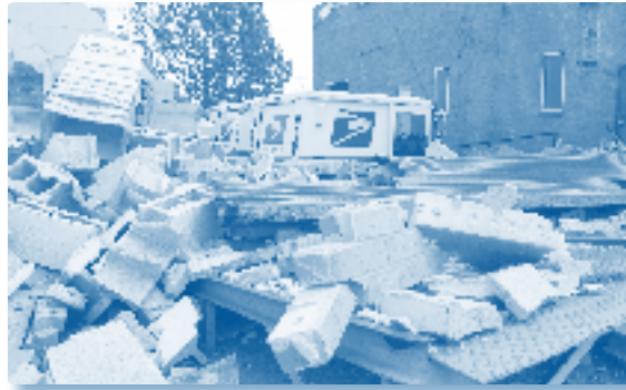
Hurricane Katrina swept into the Gulf Coast region causing an estimated $128 million in damages to the Postal Service's infrastructure.
