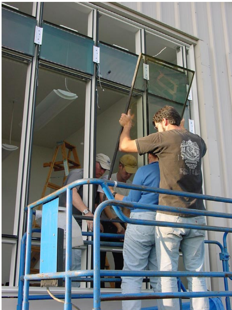
Figure 2. Installing windows
