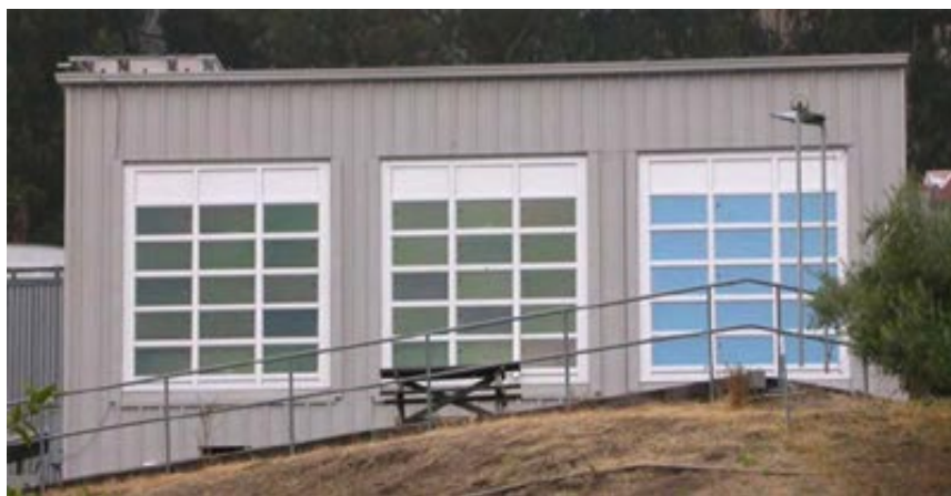
Figure 1. Picture of the Windows Testbed Facility at LBNL.
