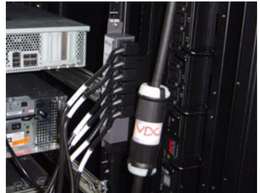
Figure 4. DC connectors need to be standardized similar to AC connectors.
