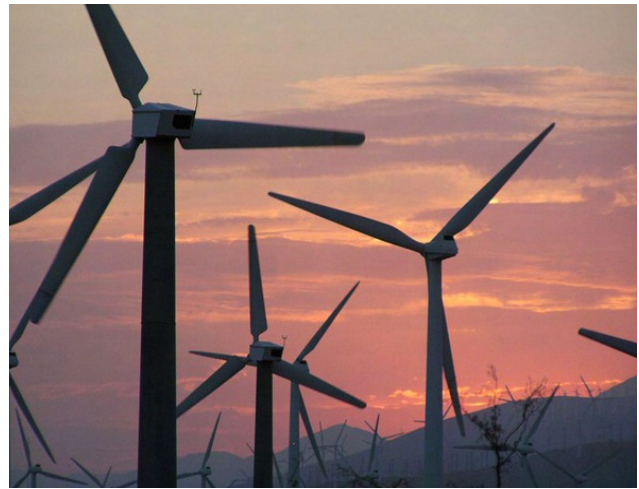
Figure 1. Eritrean officials hope to someday provide as much as 50 percent of the nation's grid electricity using wind turbines, such as these located near Palm Springs CA.
