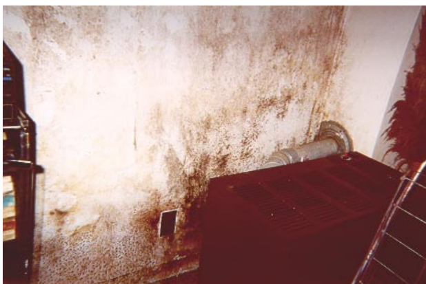
Figure 3. A living room in a San Francisco apartment in which the tenant never opened the windows (for security reasons) (Photo courtesy of San Francisco Department of Public Health)
