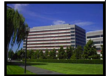
Figure 1. Three of five buildings participating in the first successful test of a multi-building internet demand-response control system: The Ronald V. Dellums Federal Building, Oakland; University of California, Santa Barbara; and Bank of America, Concord, California.
