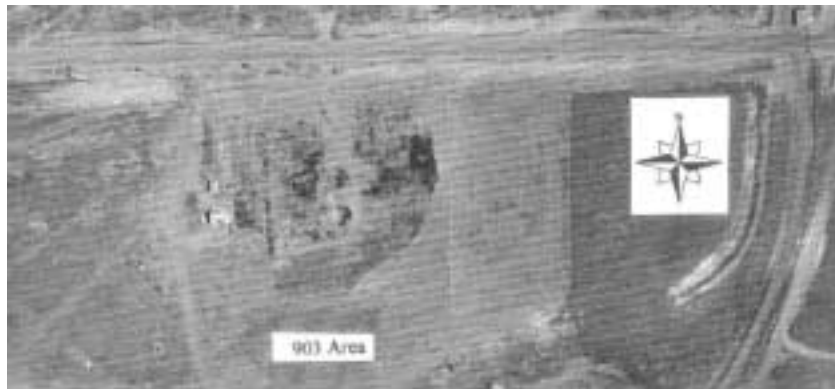
May 24, 1969. The 903 Area cleared and ready for application of cover materials.
