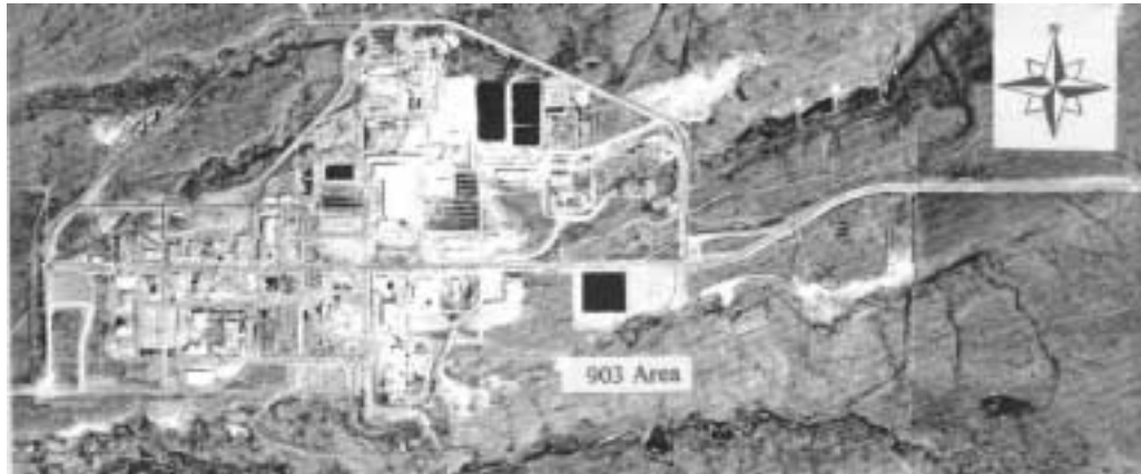
April 1970. The completed 903 Area asphalt pad (photo center).
