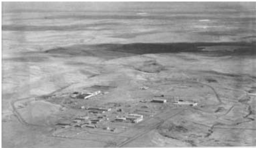
January 6, 1966. Perspective of the Plant, taken from the west.
