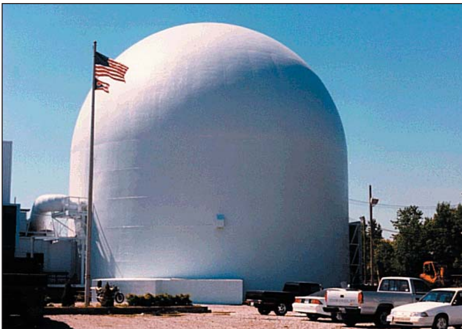
The Entombed Nuclear Reactor at Piqua, Ohio is cared for by the Long-term Surveillance and Maintenance Program.
