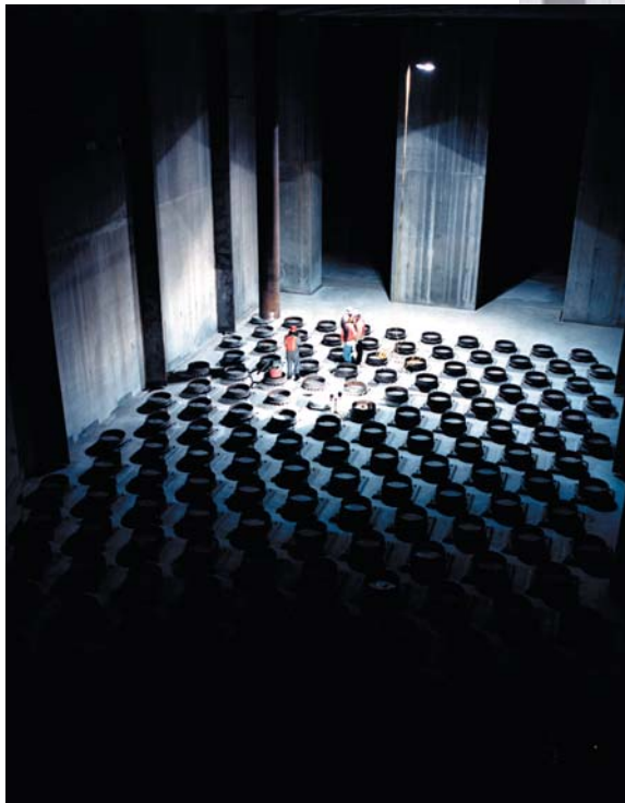
The canister storage building vault where workers are seen moving a tube to the lift site with special wheeled dollies.
