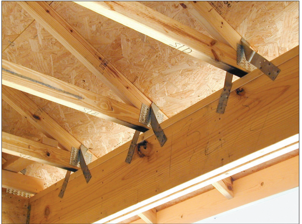
Figure 8: Hurricane Straps in a Home under Construction
