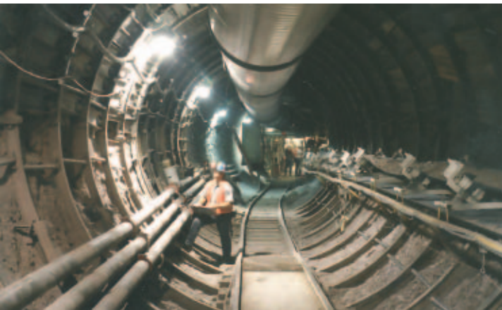
An engineer checks out a tunnel (drift) at the proposed Yucca Mountain nuclear waste repository. Sandia researchers are helping understand the mechanics of rock structure there.
