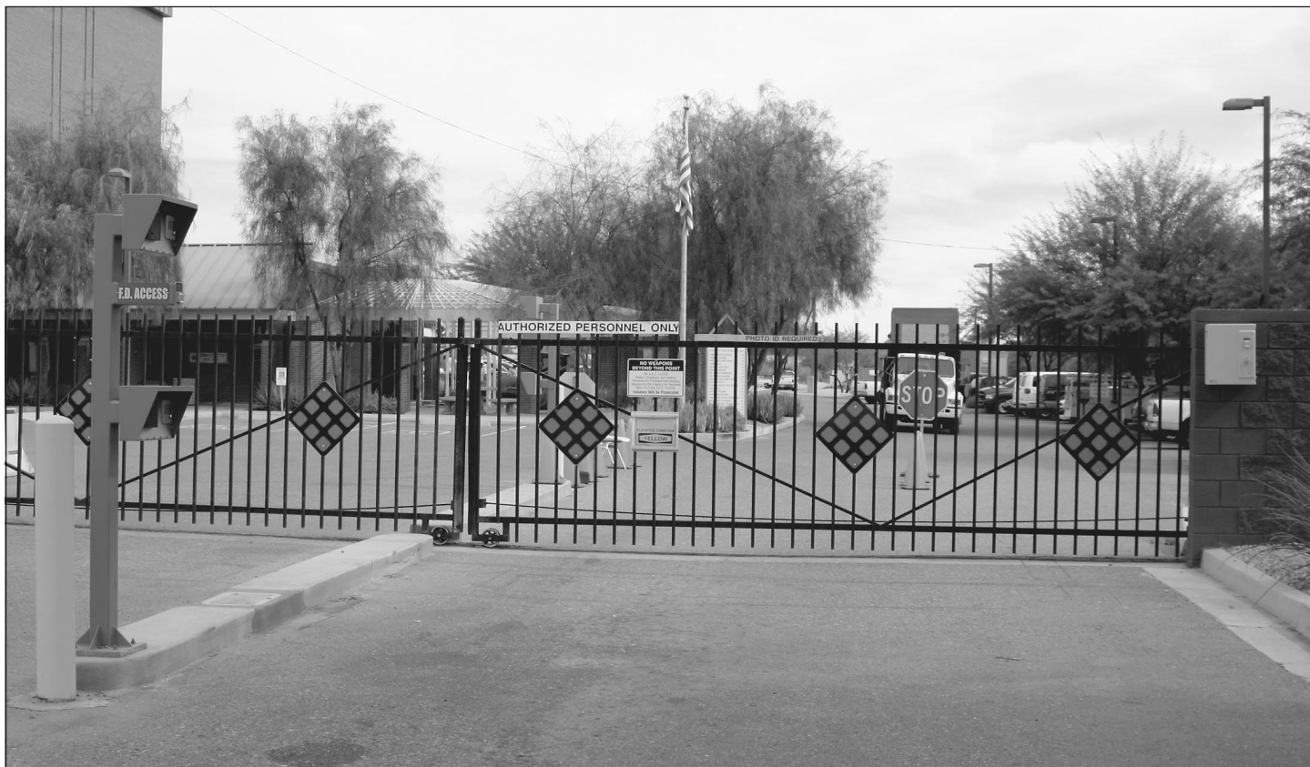
Figure 11: Electronically-Controlled Security Gate
