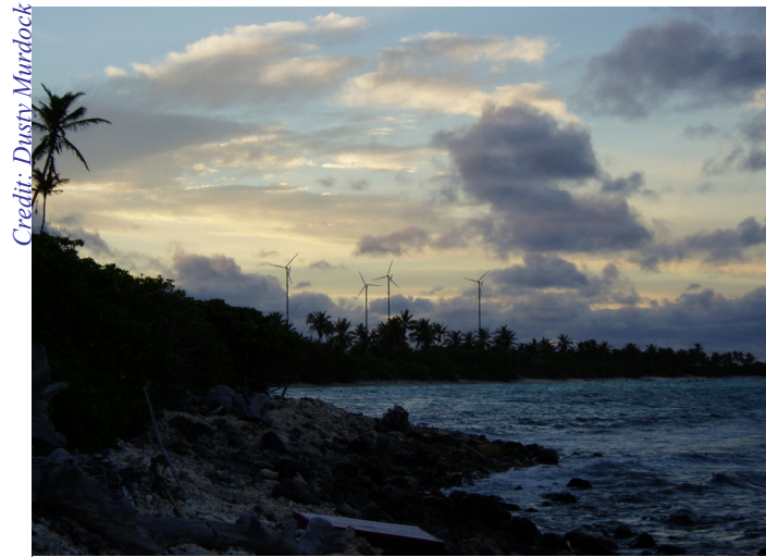
Dusty spent several weeks living on one of the remote Cocos Islands, while interfacing these four wind turbines to the power grid.
