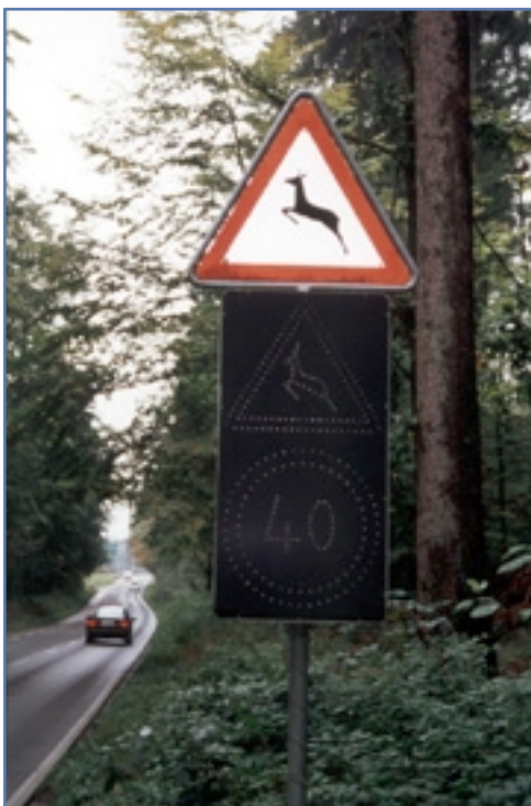
Figure 9. Fiberoptic speed limit sign, triggered when wildlife approaches the road.
