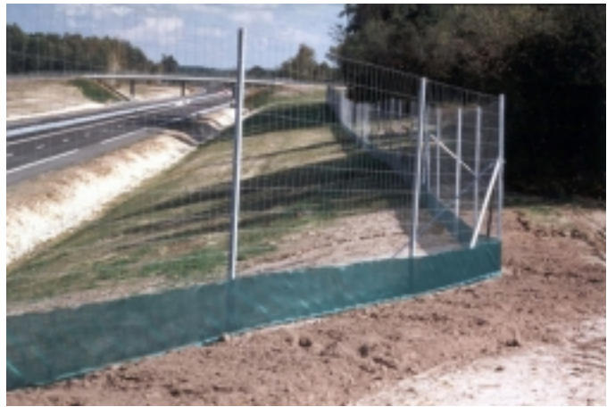
Figure 11. Fine mesh fence (the Netherlands), plastic barrier (France), plastic fabric fence (France), and rail (Germany): Applications for amphibians.
