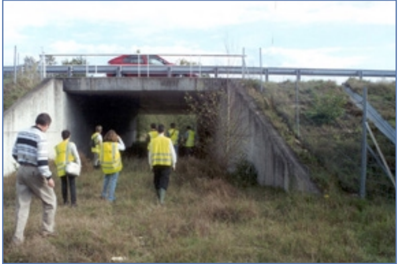
Figure 12. French box culvert overpass (3 m high and 6 m wide).
