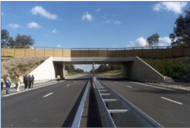
Figure 15. French overpass with board fence (15 m wide at center; 30 m wide at ends).
