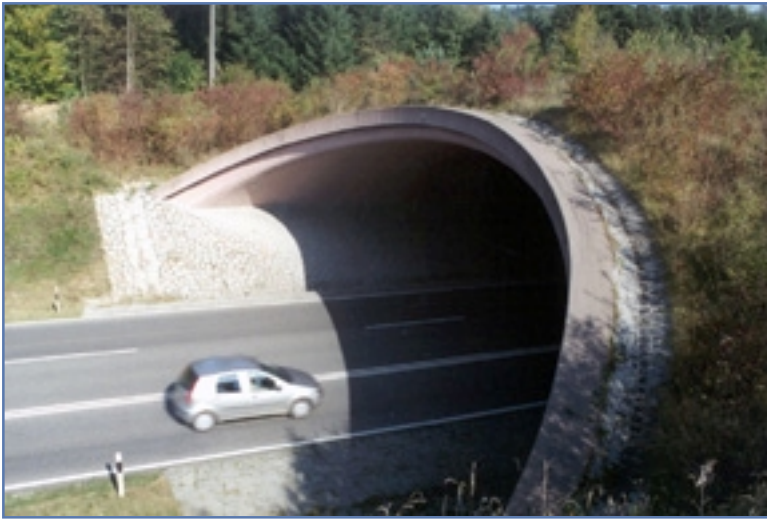
Figure 18. Swiss overpass built in 1995 with a 23-m width at center.
