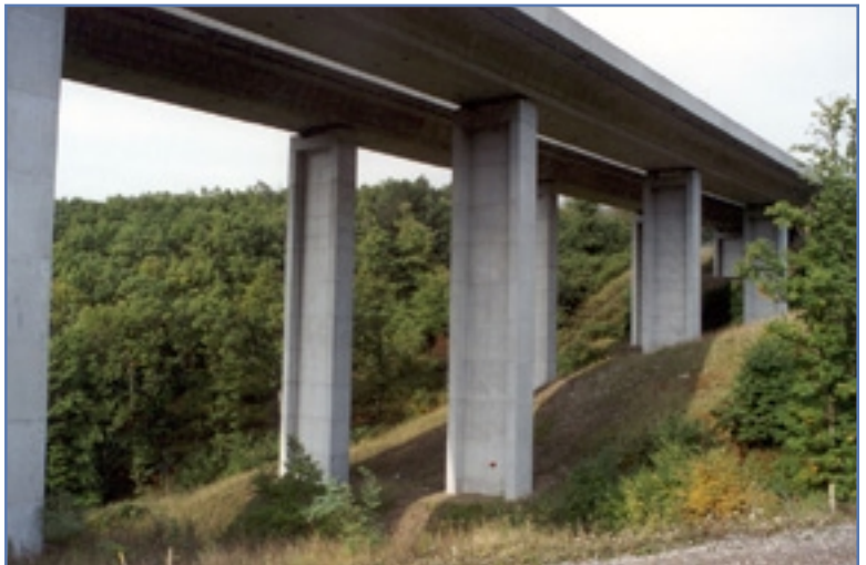
Figure 21. Slovenian viaduct built for wildlife, hydrology, and human connectivity.
