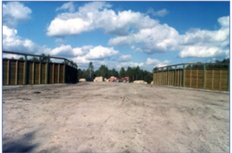
Figure 16. Board fence on French overpass to block noise and light (rocks are placed at ends to prevent vehicular use).
