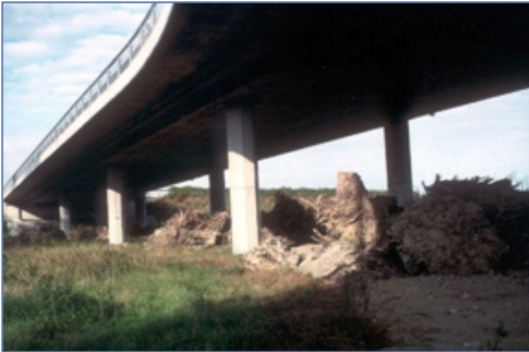
Figure 22. Swiss viaduct with stumps for small animal cover.
