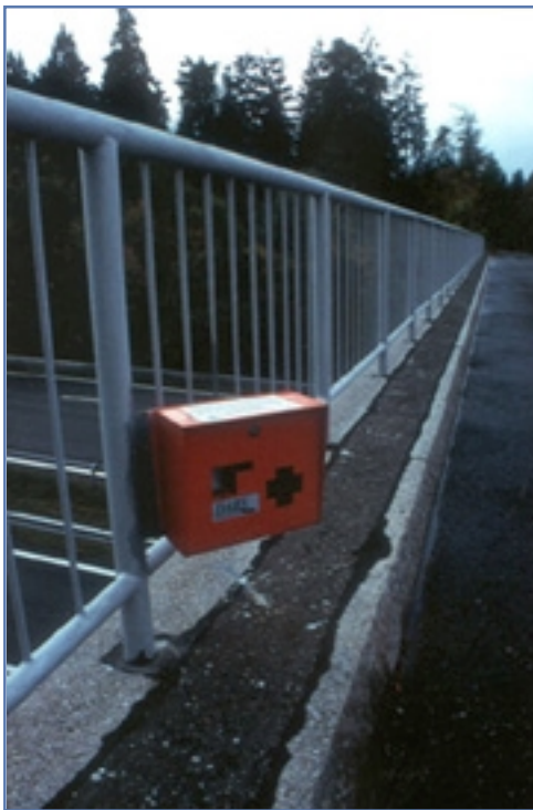
Figure 2. Infrared still camera setup with protective case on Slovenian bridge.
