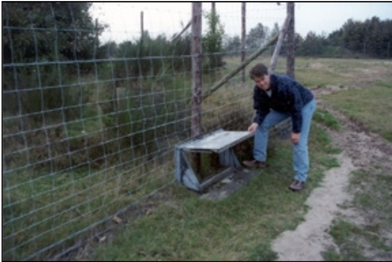
Figure 8. One-way door for small mammals on fence near Dutch overpass.
