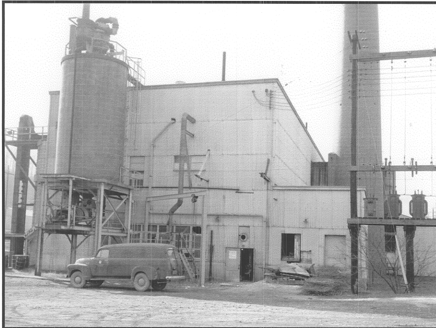
Photograph 8: Building 9401-2, one of two original Y-12 steam plants (1956). This steam plant was replaced in 1956 by a new steam plant, Building 9401-3. (Photo 100470 courtesy of the Y-12 Plant).
