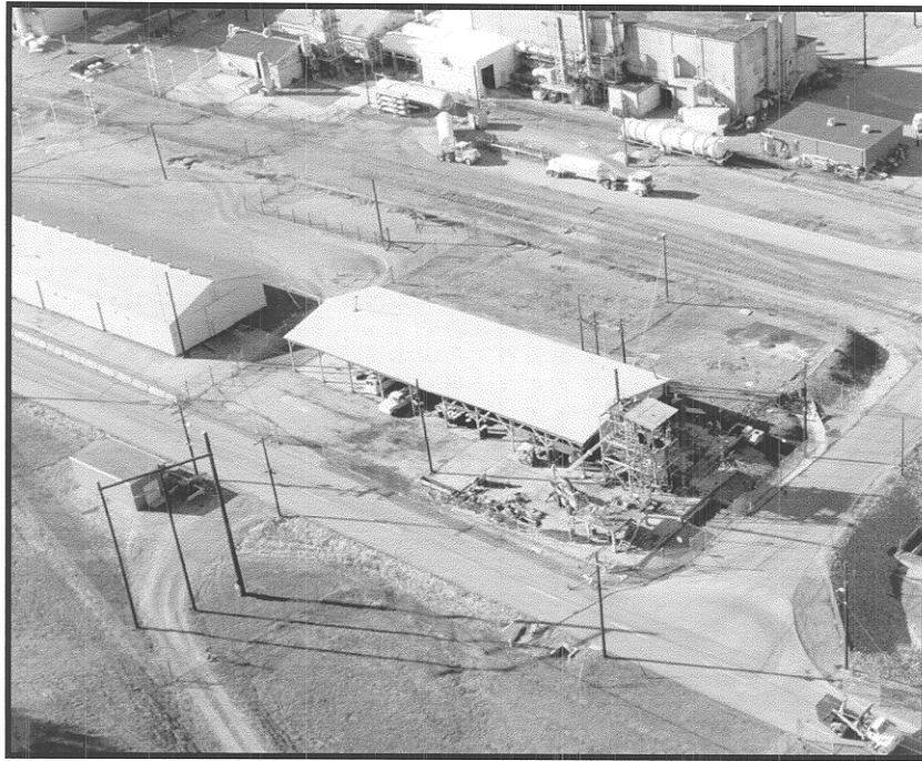
Photograph 7: Aerial view of Building 81-10, looking northwest (1983). The metal frame structure east of the building is the mercury roaster, which was dismantled after this photo was taken on November 29, 1983. (Photo 218284 courtesy of the Y-12 Plant)
