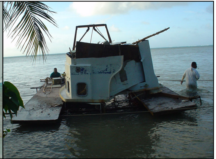
Large section of house brought to staging area on barge
