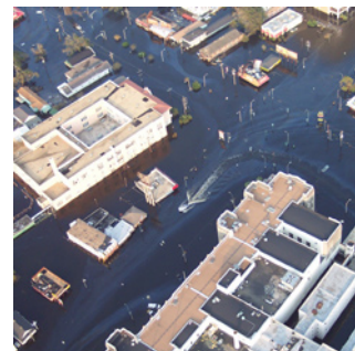
Flooded street in New Orleans, Louisiana.
