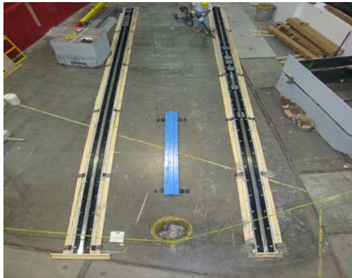
EQ-SANS tank rails have been aligned.
