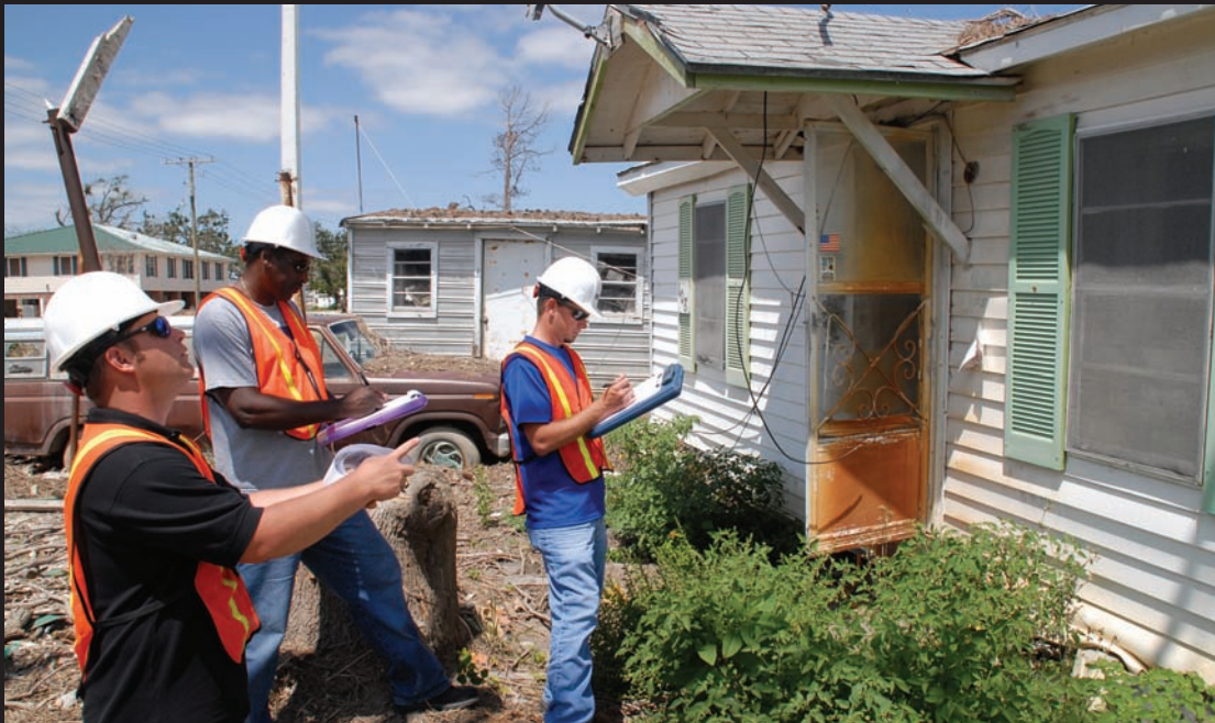
Cameron, LA, May 20, 2006—FEMA asbestos inspectors George Legere, Walter Coleman, Jr., and Rocky Craigen check for asbestos in preparation for demolition. Crews and landfill operators need to know which hazardous materials are present. (Marvin Nauman/FEMA photo)
