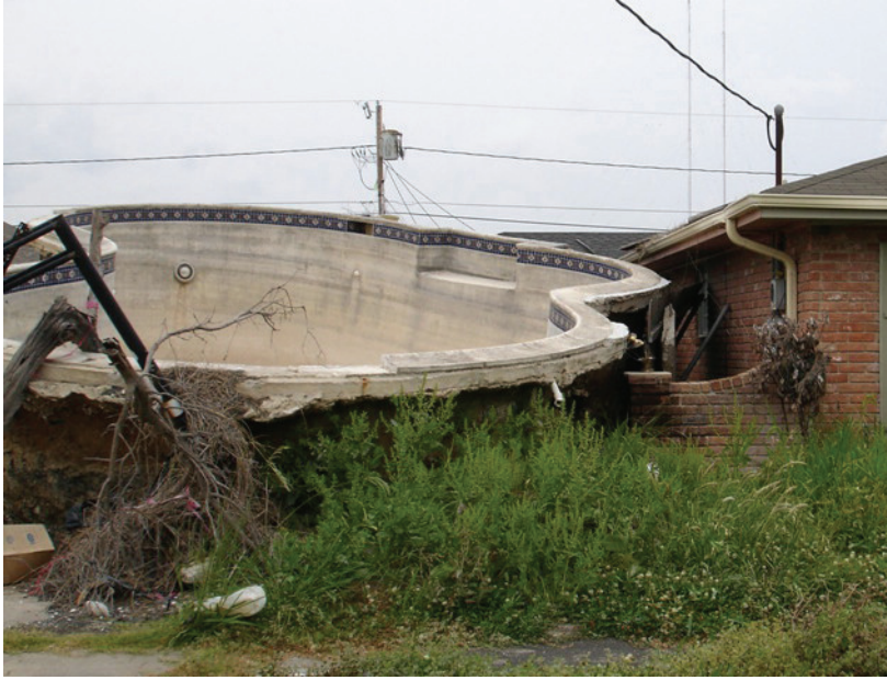
New Orleans, LA—Just outside the city, a backyard pool rests in a flood victim's front yard. (SBA photo)
