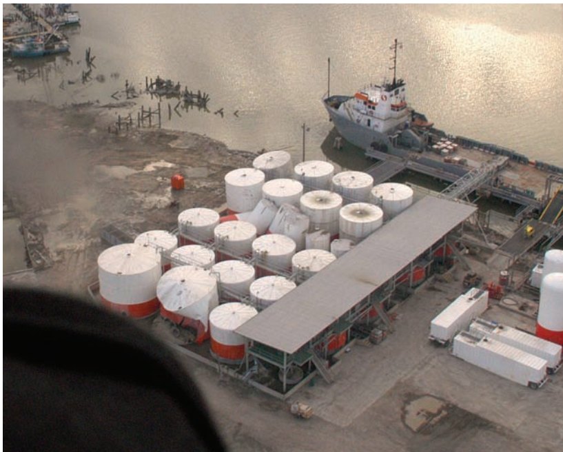
Cameron, LA—The local environment was damaged when storage tanks like these in Cameron, LA, broke and leaked and mixed with other unknown chemicals from Hurricane Rita. The EPA, funded by FEMA, undertook a massive operation to identify and clean up any hazards. (Marvin Nauman/FEMA photo)
