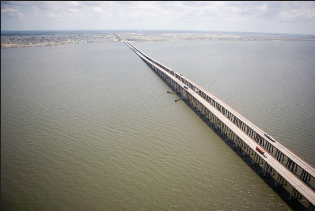
New Orleans, LA, August 14, 2006—The twin span bridge in New Orleans a year after it was badly damaged by Hurricane Katrina. The Federal Government, through FEMA, has provided billions of dollars to help rebuild infrastructure. (Ed Edahl/FEMA photo)
