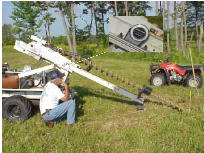
Figure N-5. Positioning the drilling boom.
