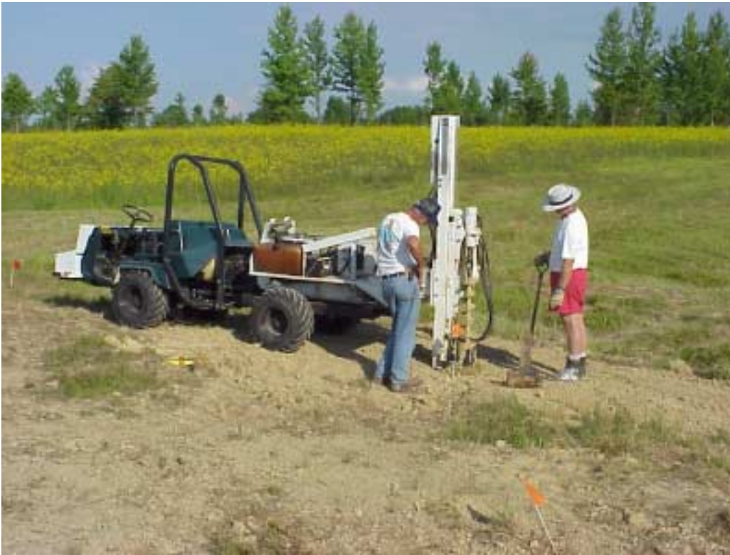
Figure N-3. Vertical drilling by Simco Earthprobe 200.
