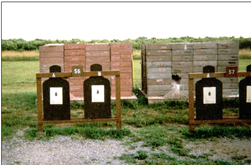
Figure II-2. SACON backstops behind 25-Meter range targets.
