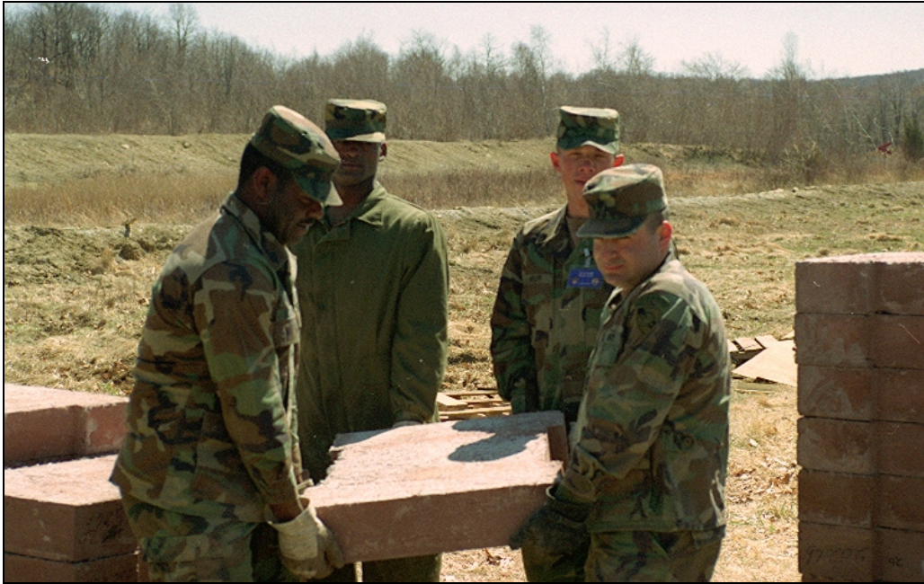
Figure IV-5. Four-man lift - 200-pound SACON block.
