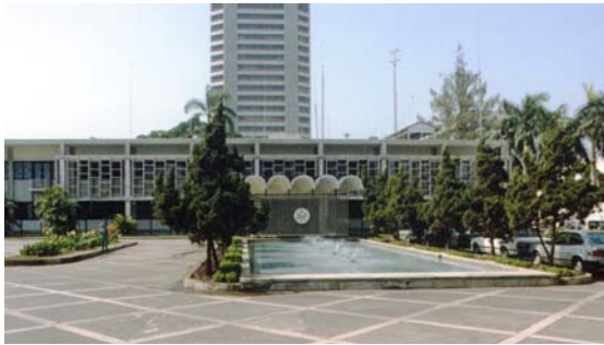
Exterior of Embassy Jakarta chancery building
