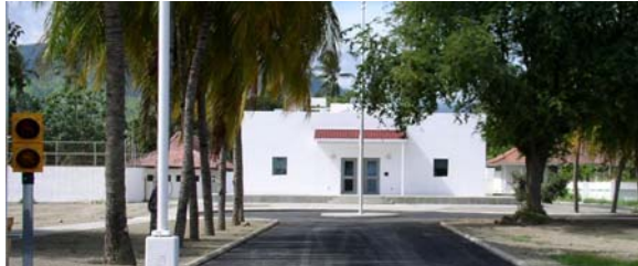
Exterior of Embassy Dili
