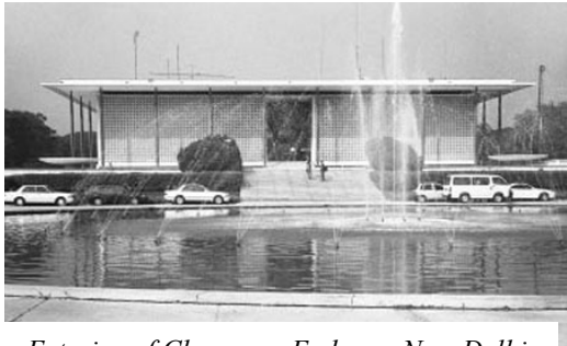
Exterior of Chancery, Embassy New Delhi
