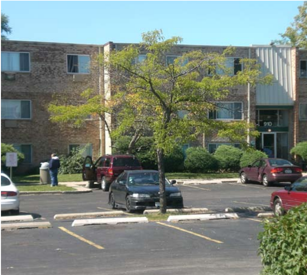
Bradford Court Apartments, renamed College Park, is a 200-unit rental housing project in Addison, Illinois.
