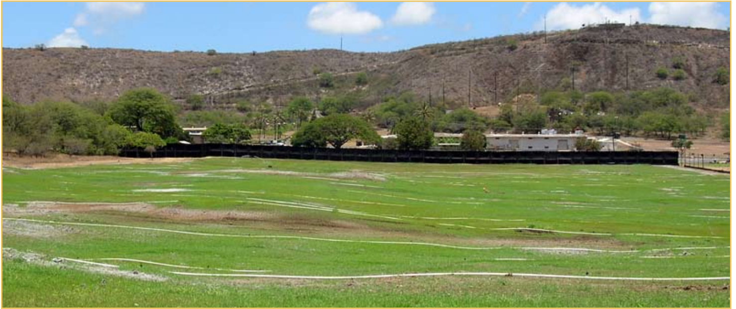
Soil removed during the restoration project was returned clean to this former rifle range. The range was hydroseeded with native grass, which was irrigated to promote growth.
