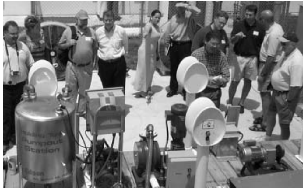
Representatives of the States Organization for Boating Access (SOBA), sewage pumpout manufacturers, and staff from Underwriters Laboratories Incorporated (UL) inspect the sewage pumpout machines that are being tested by UL. Funding for this SOBA project is being provided through the Multistate Conservation Grant Program. Photo: Kevin Atkinson, California Department of Boating and Waterways.
