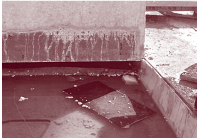
Figure 35. Leading edge of upper slab before sliding.
