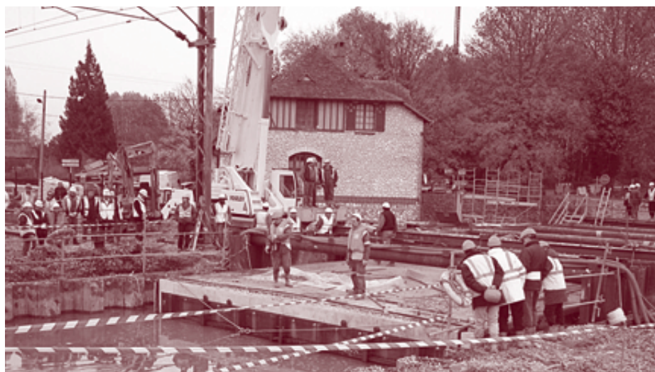
Figure 31. Floating a culvert into position.
