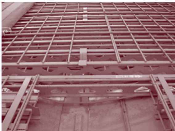
Figure 7. Hybrid steel-concrete deck system.
