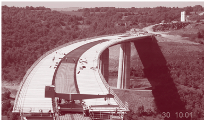
Figure 41. Full-depth precast deck panels.
