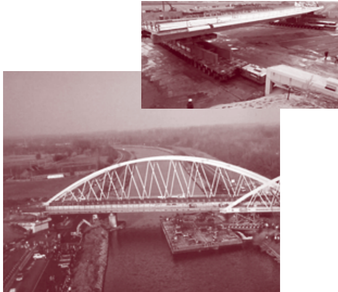
Figures 17a and 17b. Moving large bridges with SPMTs.
