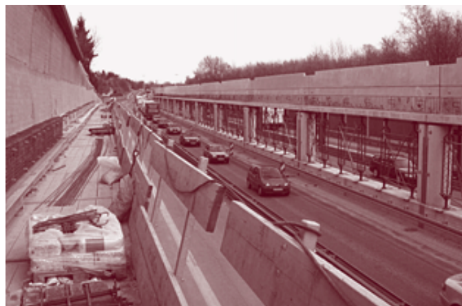
Figure 26. Construction of a noise protection gallery.
