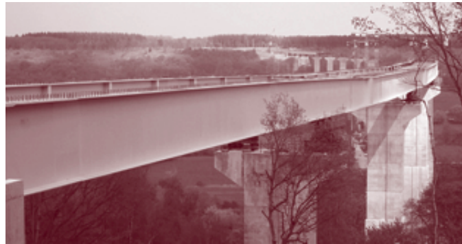
Figure 36. Risle River Viaduct under construction.
