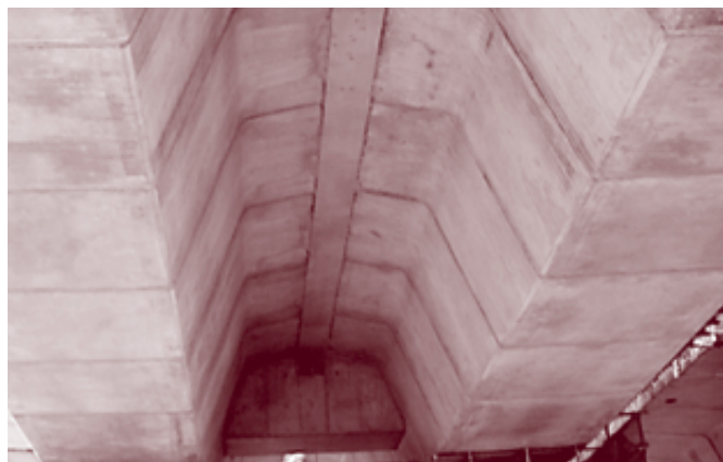
Figure 3b. Closure joint between segments.
