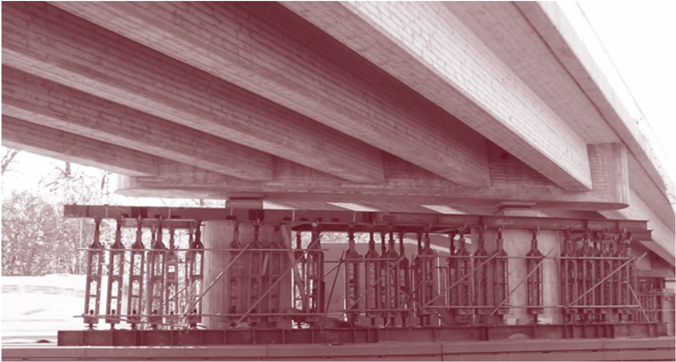
Figure 22. Temporary shoring for precast beams.
