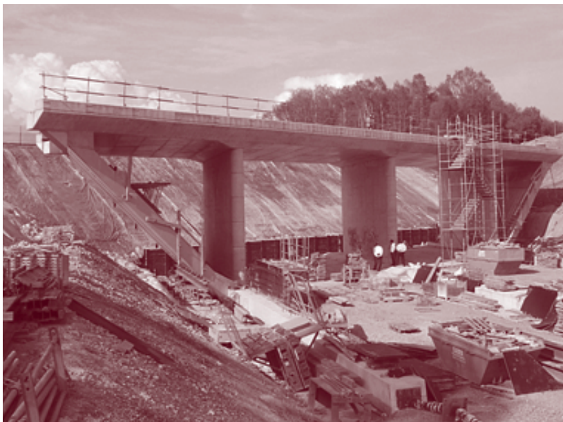
Figure 34. Railway bridge before sliding into place.
