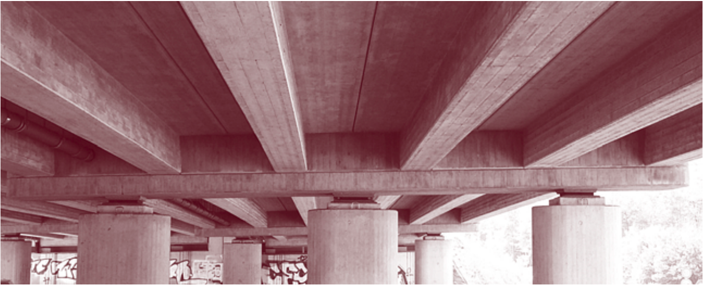
Figure 28. Precast, prestressed concrete bridge.
