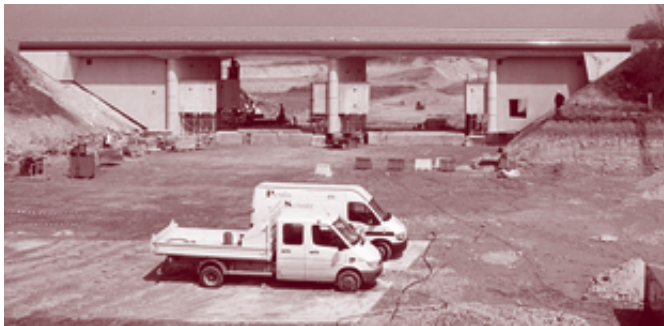
Figure 33. Railway bridge moved using SPMTs.
