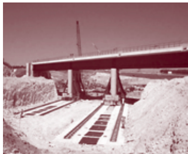
Figure 18. Skidding a bridge into position.
