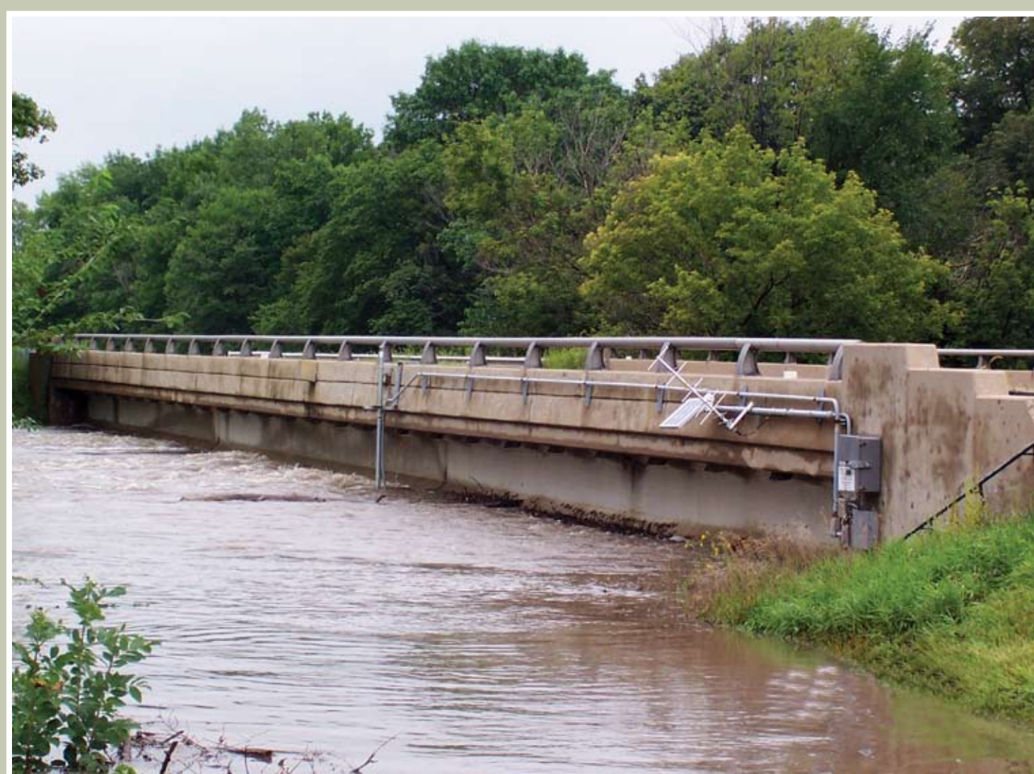
Gaging station on Aux sable Creek, Illinois
