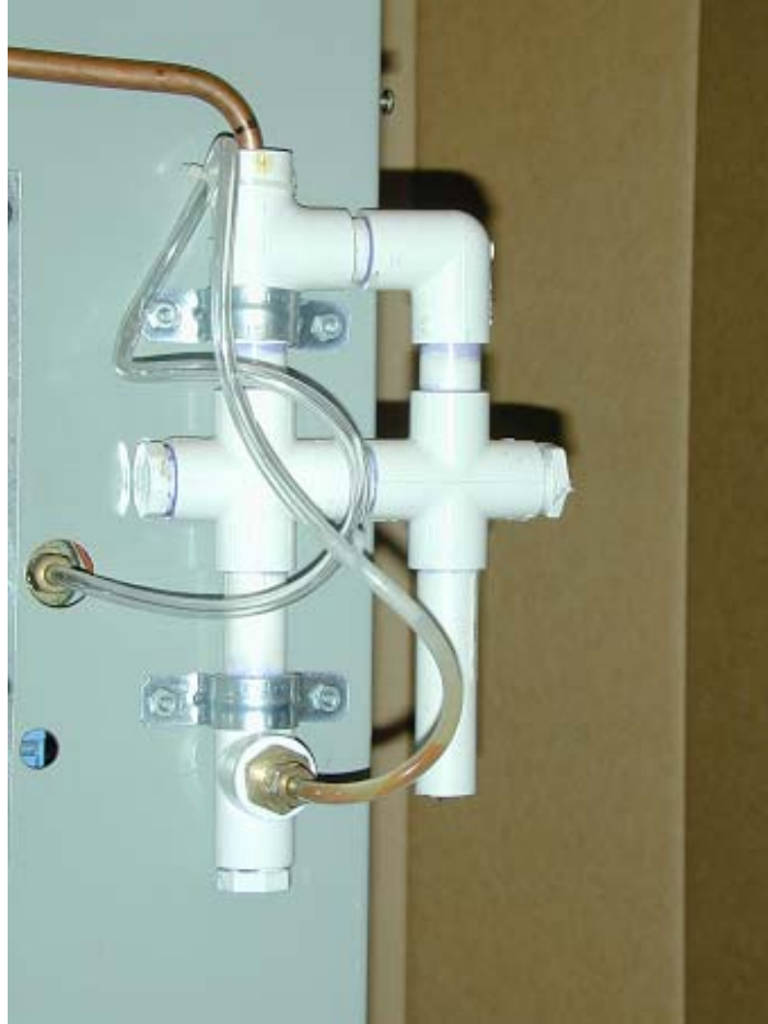
Fig. 3.3 Condensate siphon assembly.
