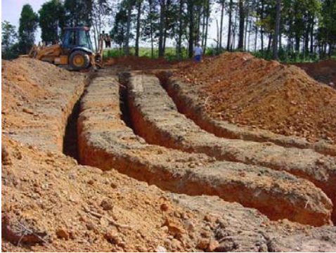
GHP trenches behind House 3.
