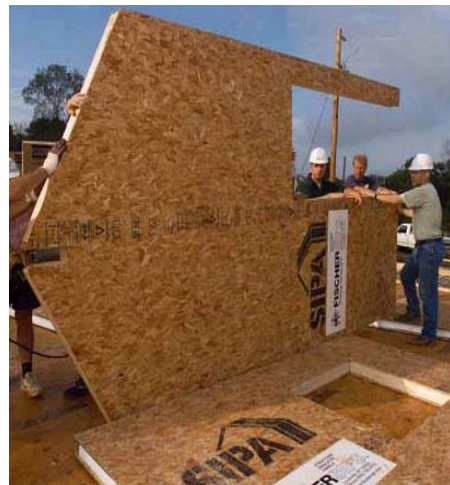
Airtight assembly of the SIP envelope is essential for energy savings.
