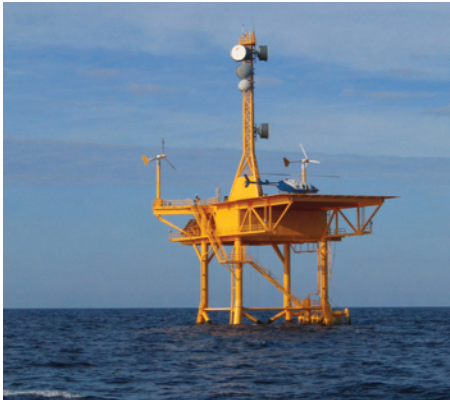
SABSOON offshore Navy towers
