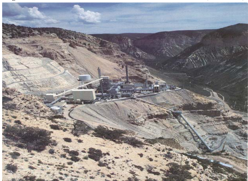
Figure 8. UNOCAL's Demonstration Plant at Parachute Creek (Circa 1990)
