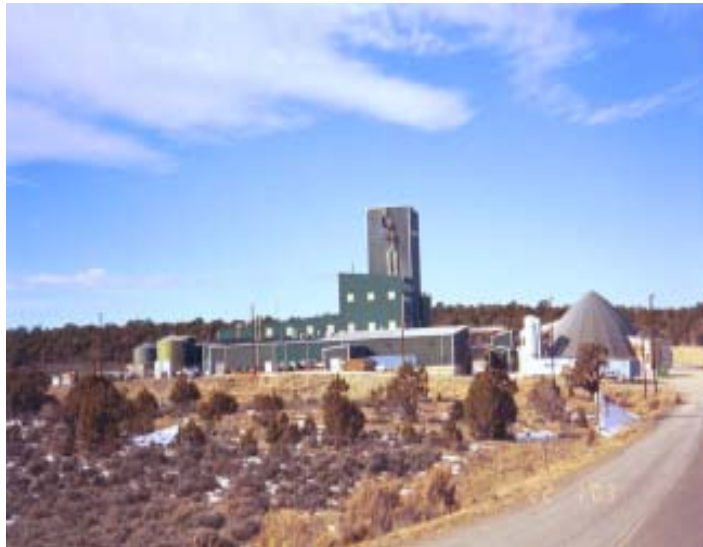
Natural Soda's Current Sodium Plant
