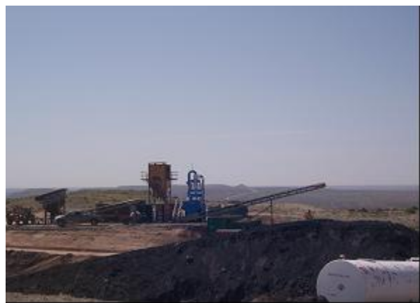
TME's Oil/Tar Sands Pilot Plant
